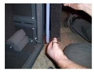
2. Lightly pull the foam taut to the bottom bracket
