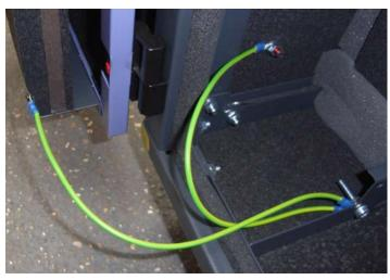
For 8210 and 8250 models the same process applies but Earthing Wires are only fitted to the front doors and side panels.
